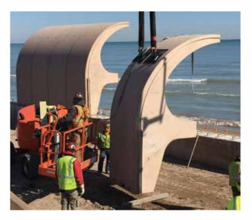
Considering the powerful waves crashing against the wall and the freeze-thaw environment of Lake Michigan, designers knew that precise placement of epoxy reinforcement, embedded stainless steel angles, and hot dipped galvanized/epoxy connectors within the high strength concrete would require a precaster that had a long-standing history of top-notch performance.
