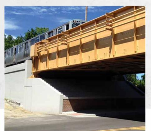
Wingwalls are adjacent to the abutment and act as small retaining walls to further support the embankment. Typical on-site CIP construction for these components is a slow process.To decrease on-site construction time, the solution is to precast these items in an off-site plant. The pieces can then be trucked to the site and quickly erected and fastened using one, or a combination, of the innovative connection options available for precast.
